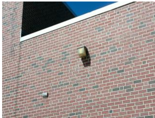
Aged Building Mounted Light
