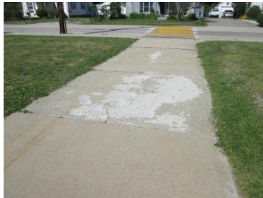
Spalled Sidewalks
