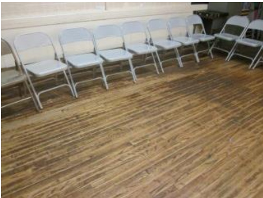
Worn Wood Stage Floor
