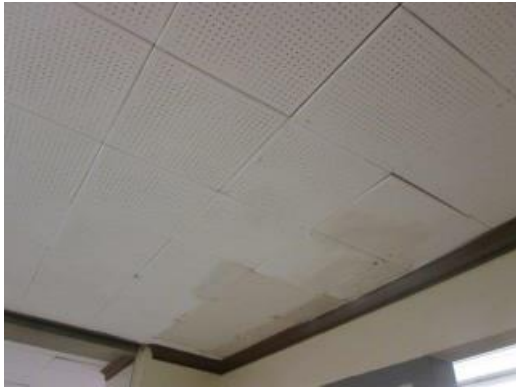
Adhered Tile Ceiling
