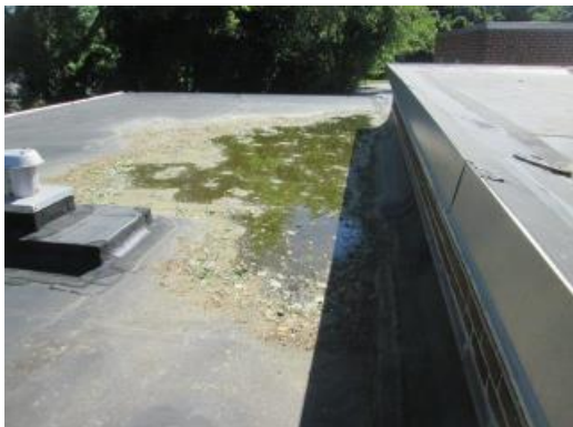
Main Building Roof
