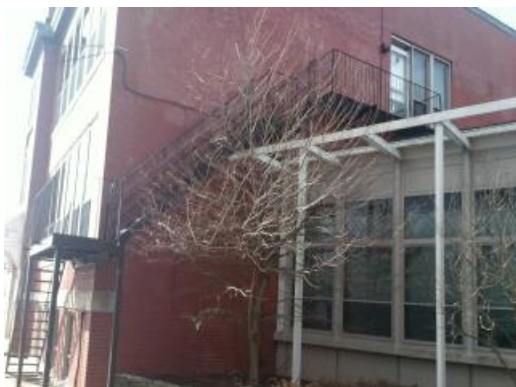
Fire Escape From Second Level
