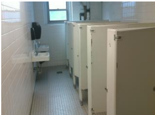
Addition Girls Restroom
